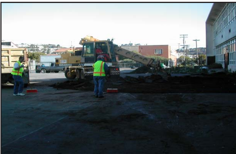
Site of the Redwood Reading Circle before planting.
